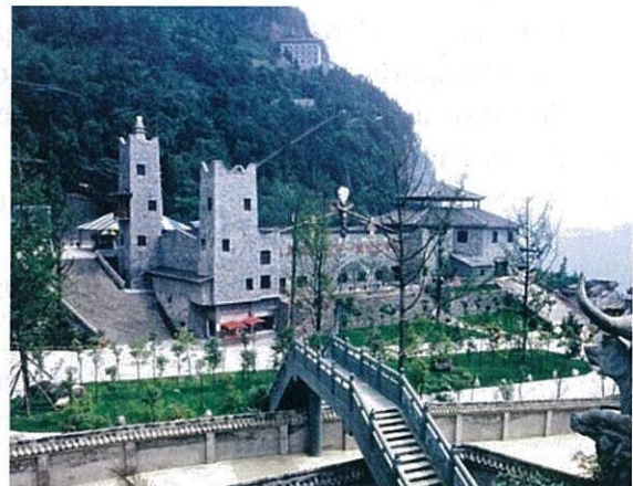
Photo 13: Reconstructed Jiuhuangshan Scenic Spot
