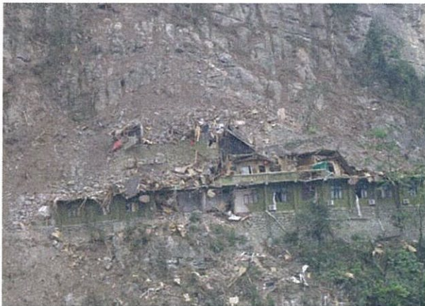
Photo 12: Damages of Jiuhuangshan Scenic Spot
